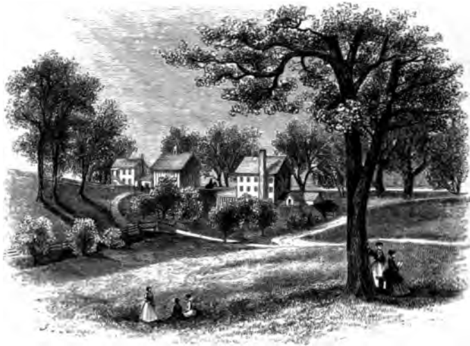
THE PUMP-HOUSE AND ITS SURROUNDINGS.
